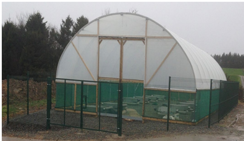
Storage facility with 12 tanks, vented sides simulating slatted shed
